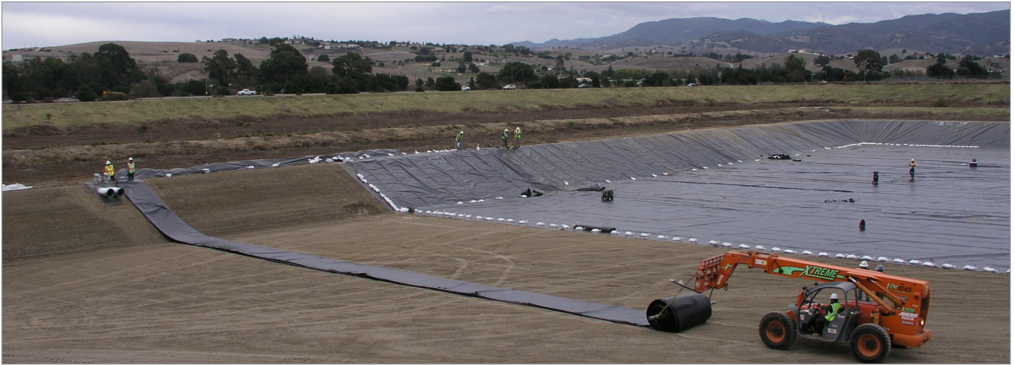
AquaMaster 45L being installed in large panels
