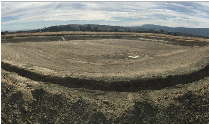
Site ready for installation of liner
