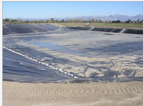
Completed pond ready for water
